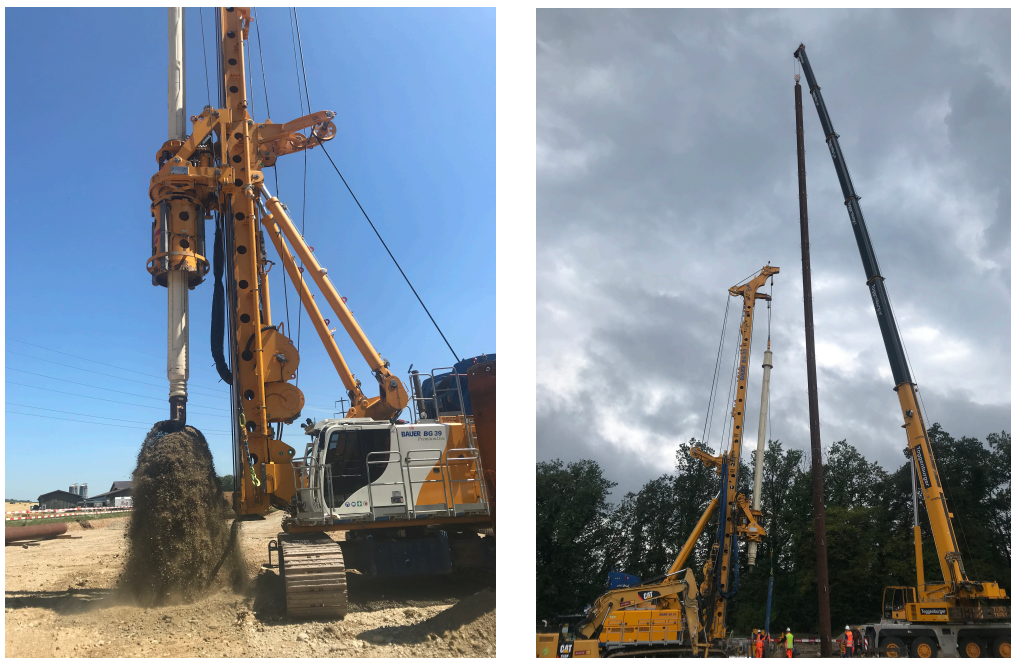
Fig. 3-1: Drilling (left) and installation (right) of the conductor
