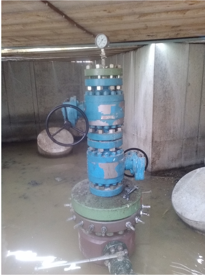
Fig. 3-14: Wellhead installed after finishing drilling operations
