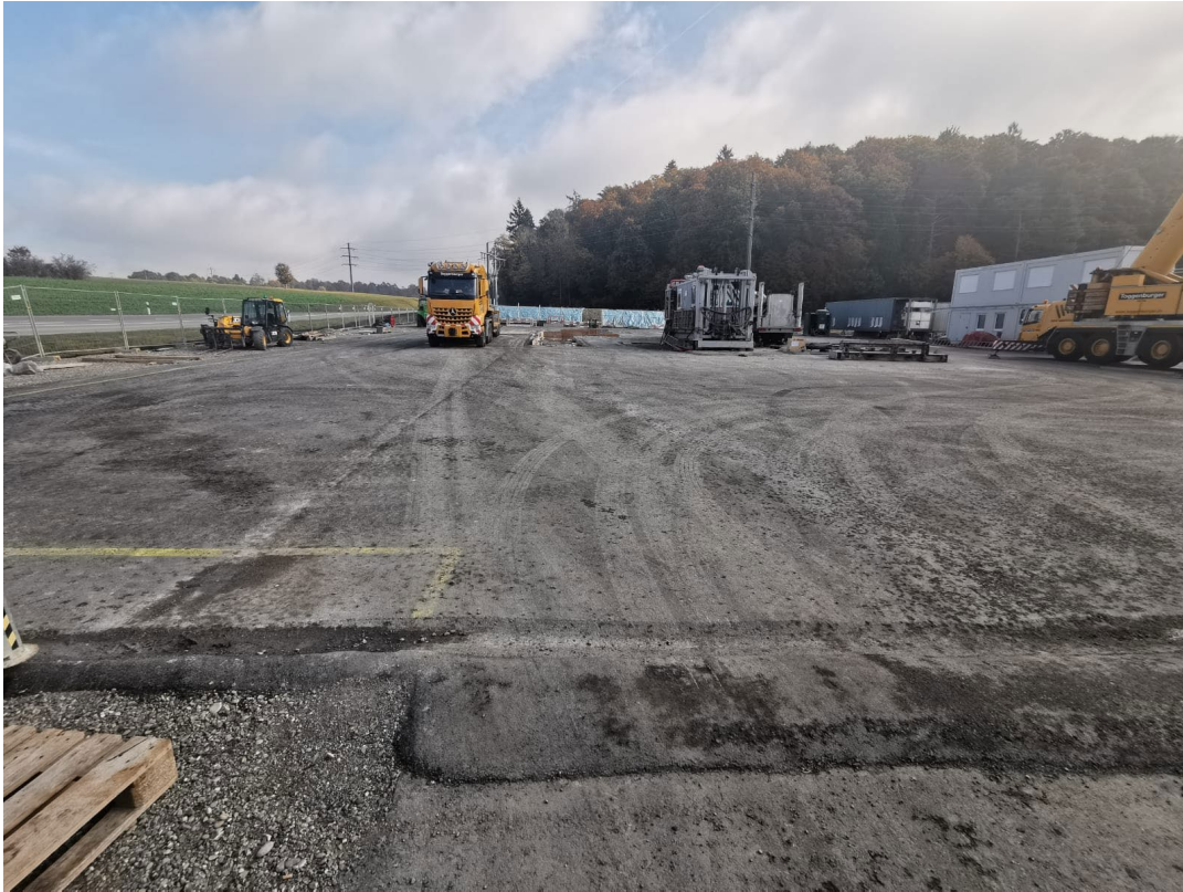
Fig. E-5: Paving the site
