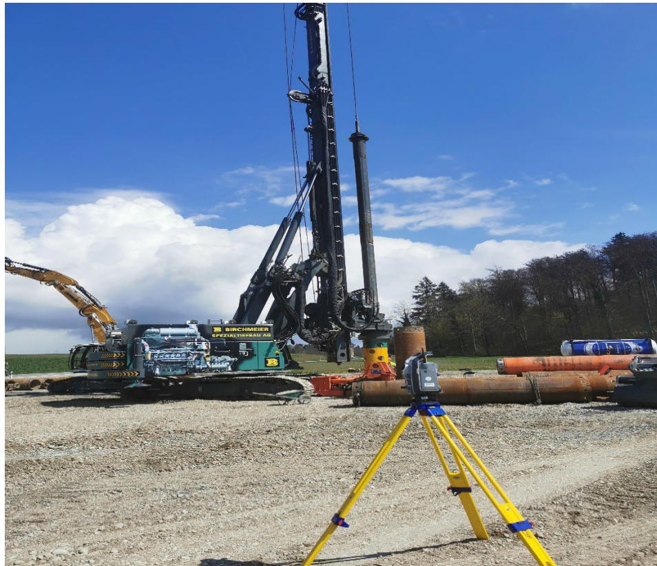
Fig. 3-2: Drilling the hole for the 13 \frac{3}{8} " standpipe
