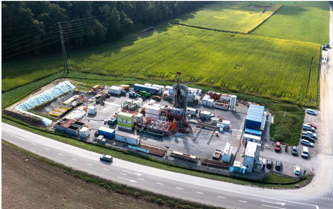
Fig. 3-1: Picture of the drill site
