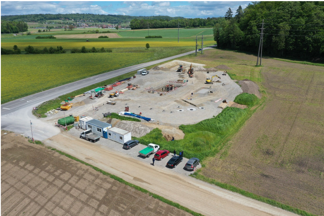
Fig. E-4: Construction of well cellar
