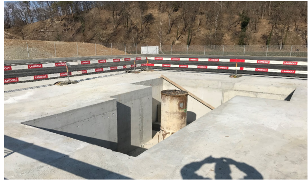
Fig. C-2: Drill cellar with standpipe
