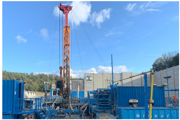
Fig. C-4: Rig and noise reduction walls
