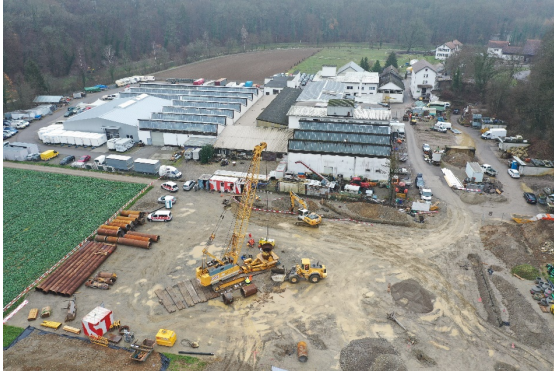
Fig. C-1: Site construction / construction of standpipe
