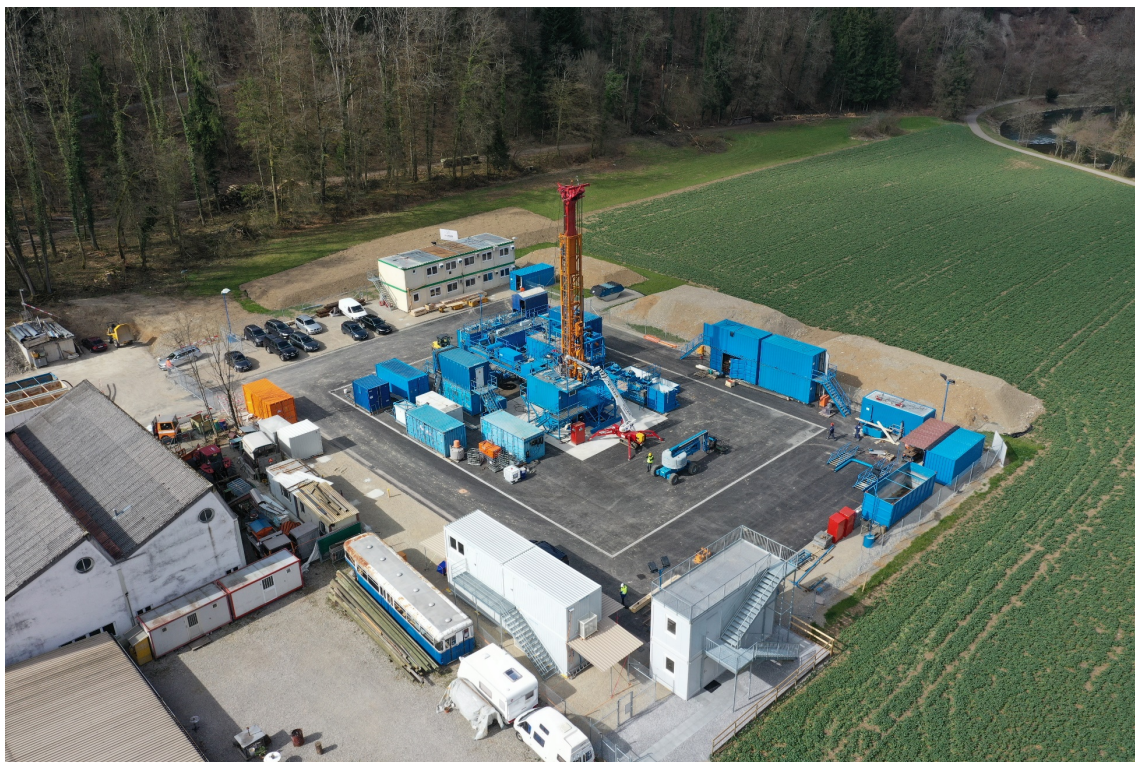
Fig. 2-1: Drill site after rig up of the Daldrup drilling rig
