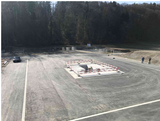
Fig. C-3: Site, ready for installations of drilling equipment
