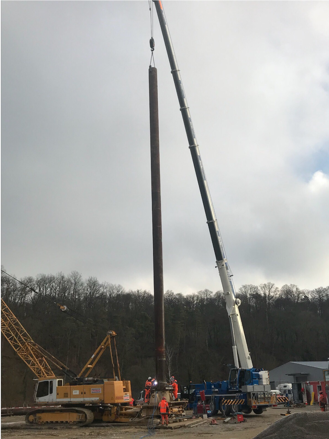
Fig. 2-2: Run in hole (RIH) 30" standpipe (welding)
