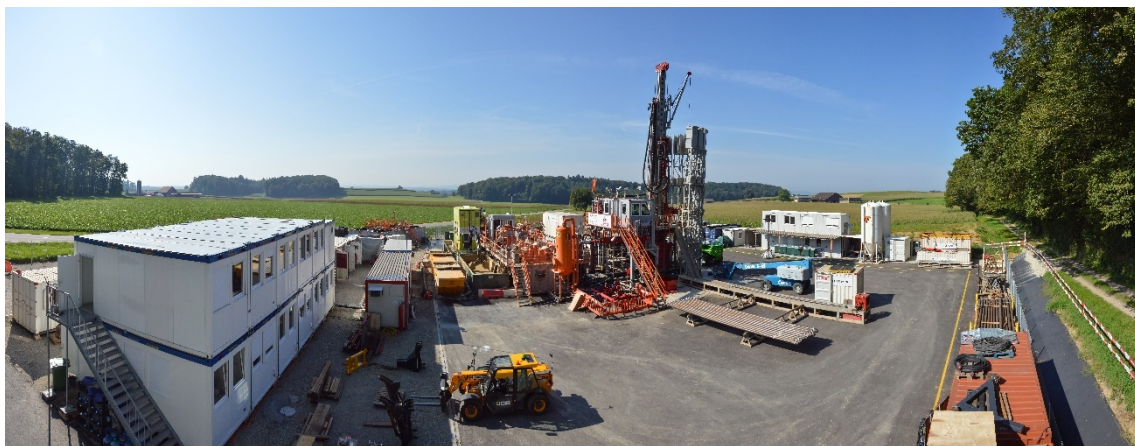
Fig. 2-1: Trüllikon drill site with rigged up Marriott's rig 16
