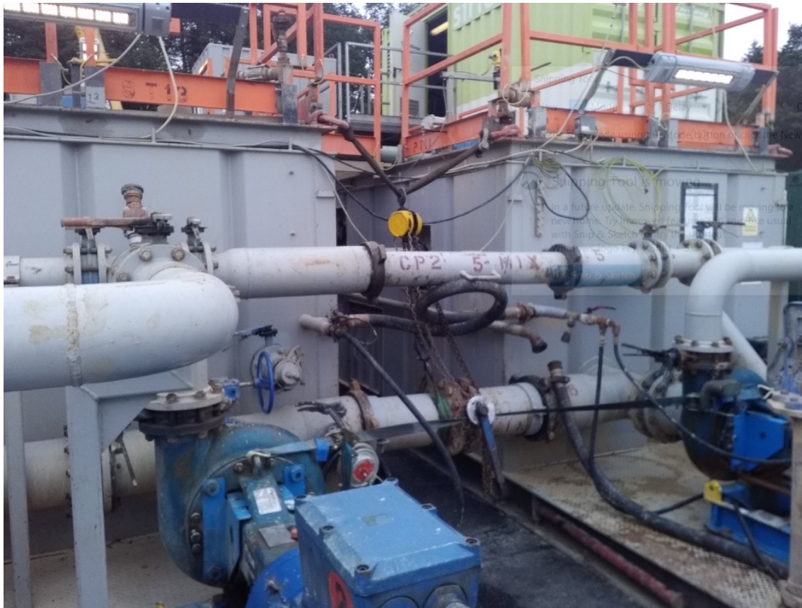
Fig. 4-1 Connection between active and mix tank
