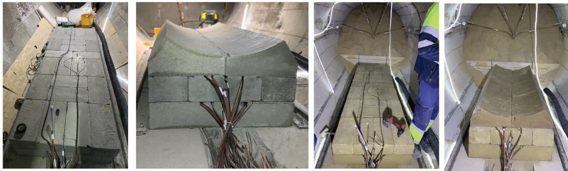
Fig. 5-2: Impressions from the construction of the bentonite block pedestal
