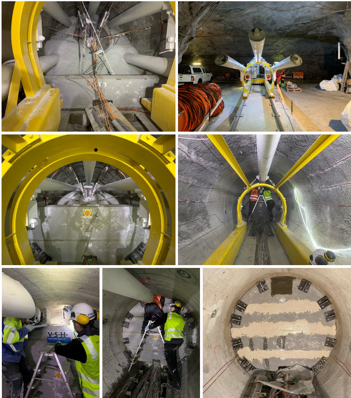
Fig. 5-9: Impressions from the backfilling procedure behind the retaining wall
