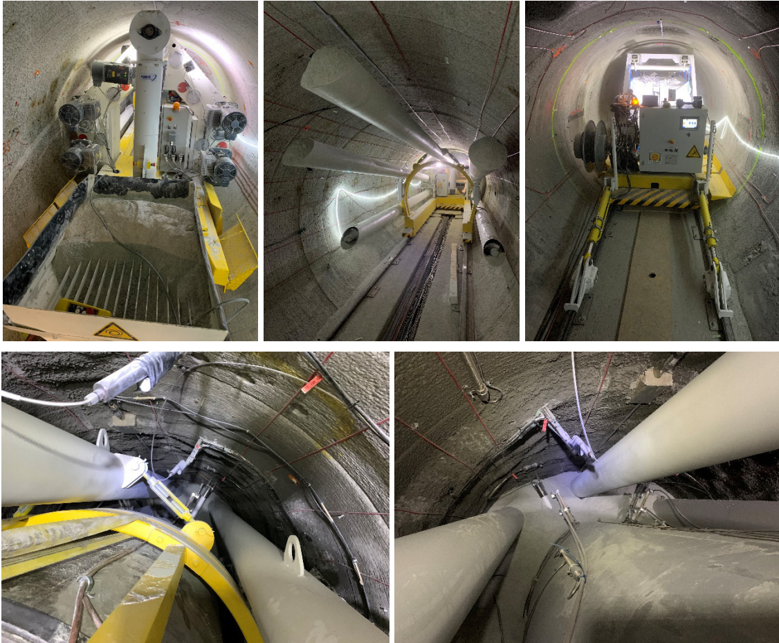
Fig. 5-4: Impressions from backfilling
