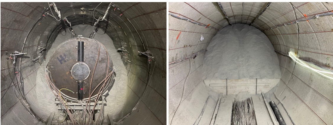
Fig. 5-5: Typically backfilled slopes around the heater (left) and without the heater (right)
